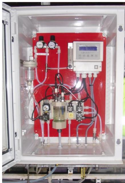
Picture to the left is the PH-1500 analyser after one year of operation in the hydrochloric acid nickel matte leaching process.
